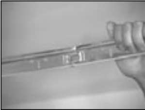
Join sections of main beam
