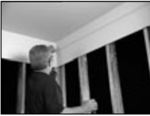
Mark desired height for new ceiling
