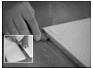
Tegular-edge border panels may require field cutting. Cut border panels face up
