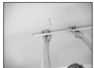
Install first main beam
