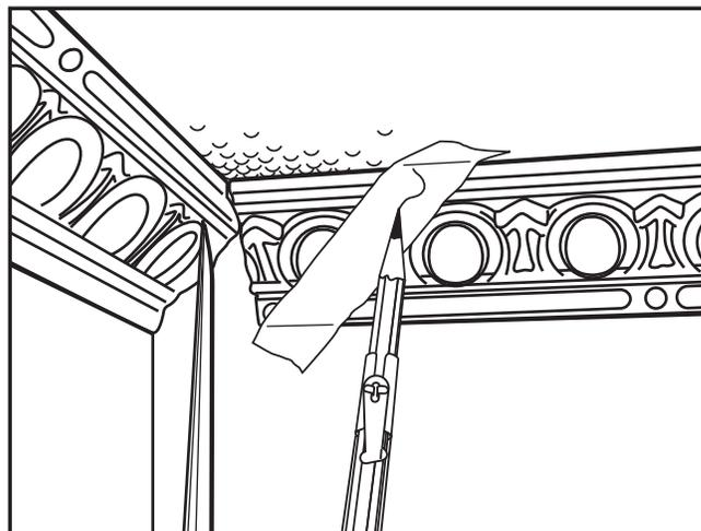
Cut along the scribed line and test fit the coped cut. You may have to make some minor trim cuts to make the parts fit. Once the coped end fits, you can use it as a template to mark a length of cornice for installation. If you are using bare steel cornices that will be painted, you can use putty to fill in any bad fitting joints.
